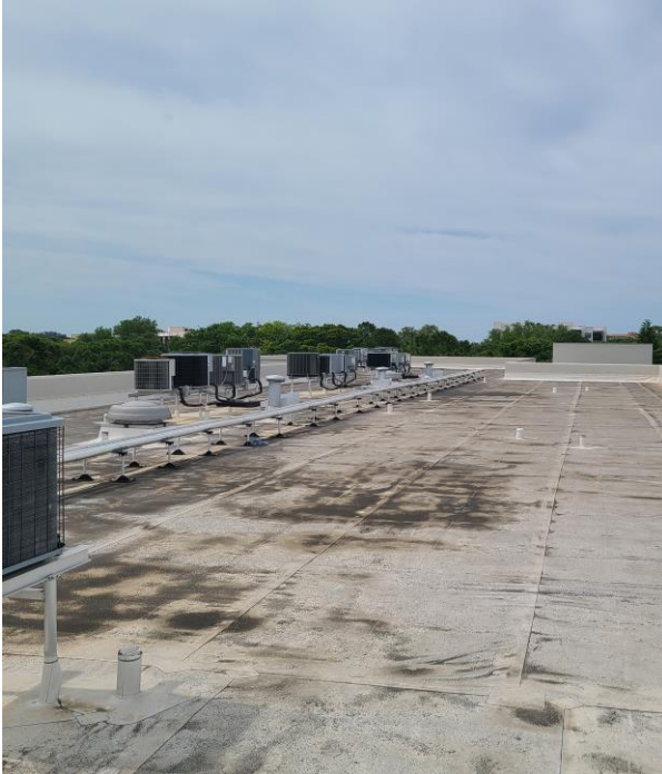
ROOF COVERING (SECTION 2)
