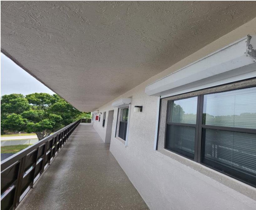
WINDOW PROTECTION / SOME UNITS (SECTION 7)
