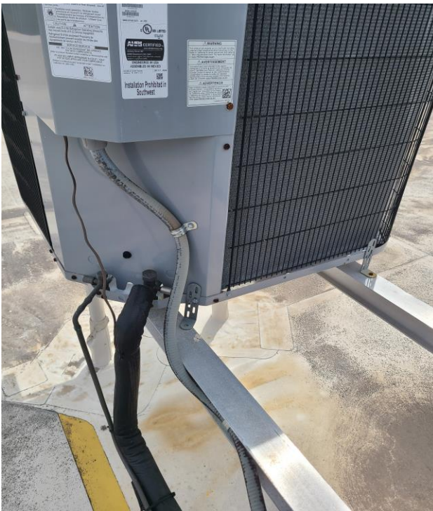
HVAC CONDENSERS, ALUMINUM STANDS ANCHORED TO CONCRETE SLAB. HVAC CONDENSERS SCREW DOWN TO ALUMINUM STANDS.
