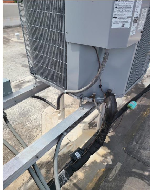
HVAC CONDENSERS, ALUMINUM STANDS ANCHORED TO CONCRETE SLAB. HVAC CONDENSERS SCREW DOWN TO ALUMINUM STANDS.
