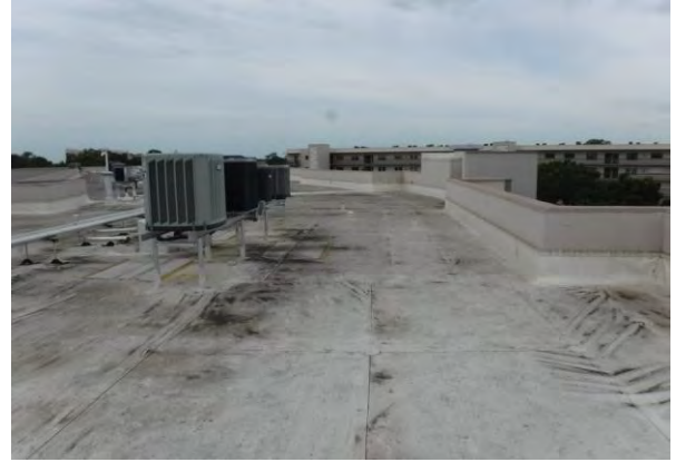
12 Roof System Overview
