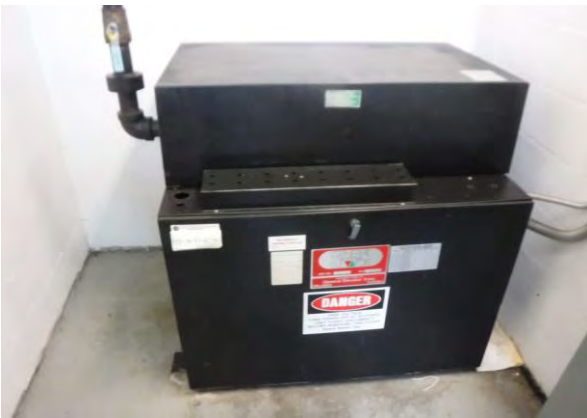
21 Elevator Motor and Controls
