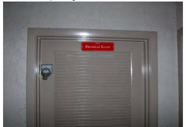
54 Utility Door Overview
