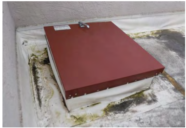
58 Roof Hatch Overview
