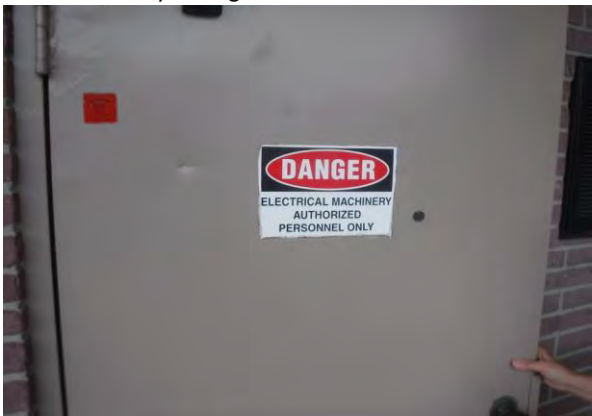
53 Utility Door Overview
