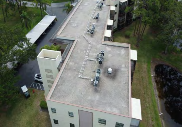
9 Roof System Overview
