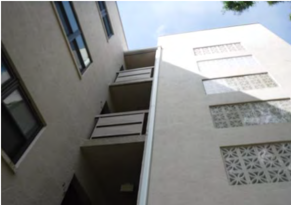
13 Building Paint Overview
