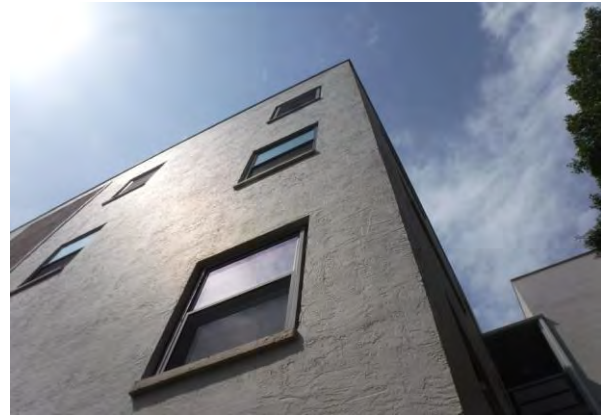
14 Building Paint Overview
