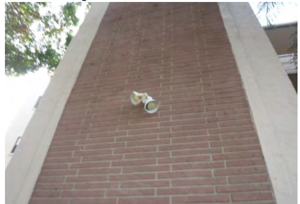
16 Building Paint Overview
