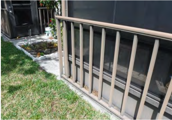
51 Balcony Railings Overview
