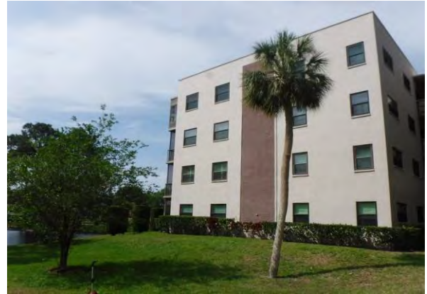
4 Left Side of Building
