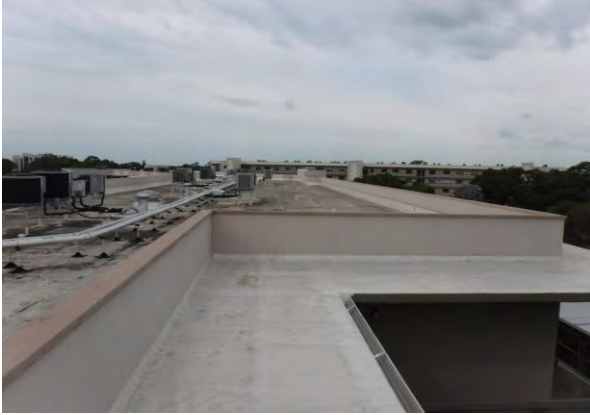
11 Roof System Overview
