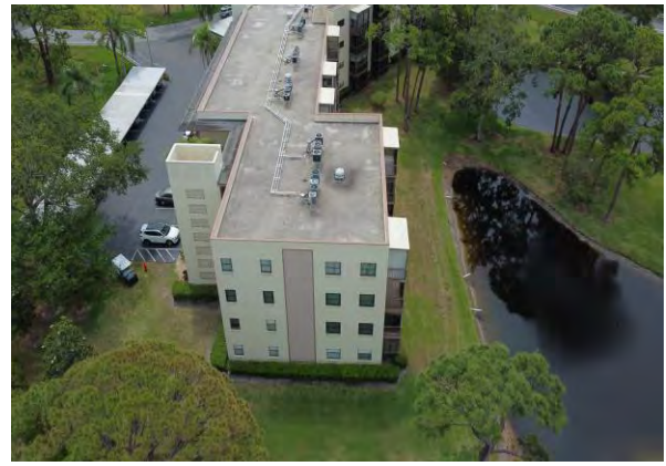
2 Right Side of Building
