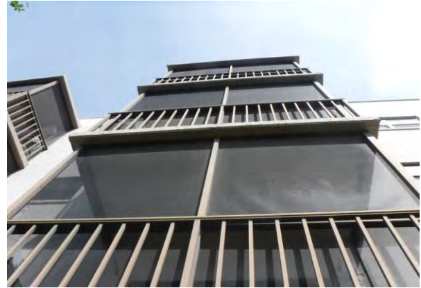
52 Balcony Railings Overview
